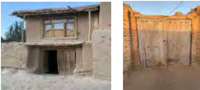
Fig 10.The exit gate of local houses
