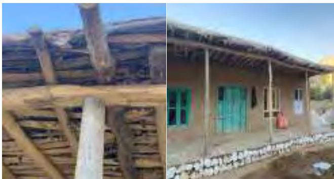
Fig 13."Megaron" adobe houses in Faryab or gallery in front of the rooms in house
