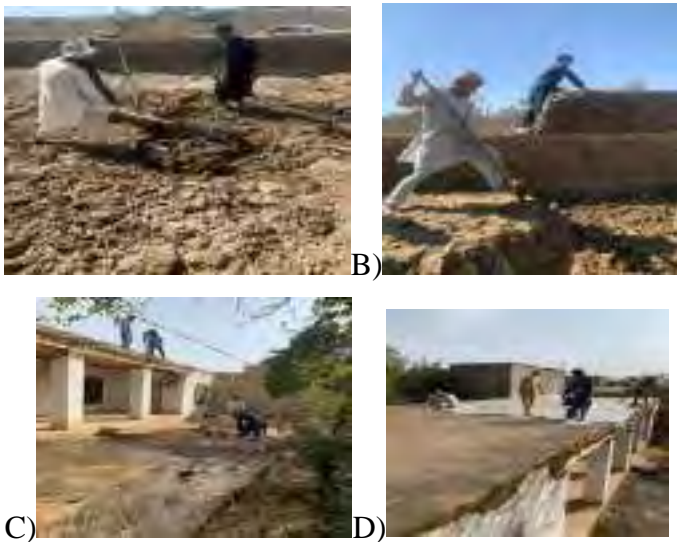
Fig 15.(A-B)Soil with water (pakhsa) for making of wall (C-D)soil ,water and straw for (khagil)covering the roof primary materials of residential house
