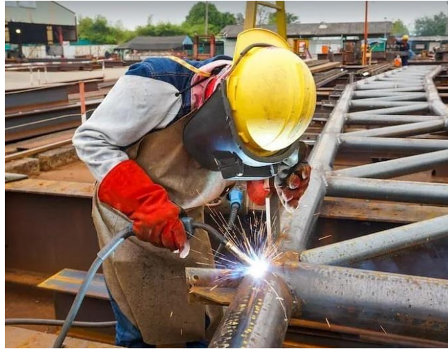
Figure 2. FluxCored Arc Welding (FCAW) Method (fractory.com, 2023).
